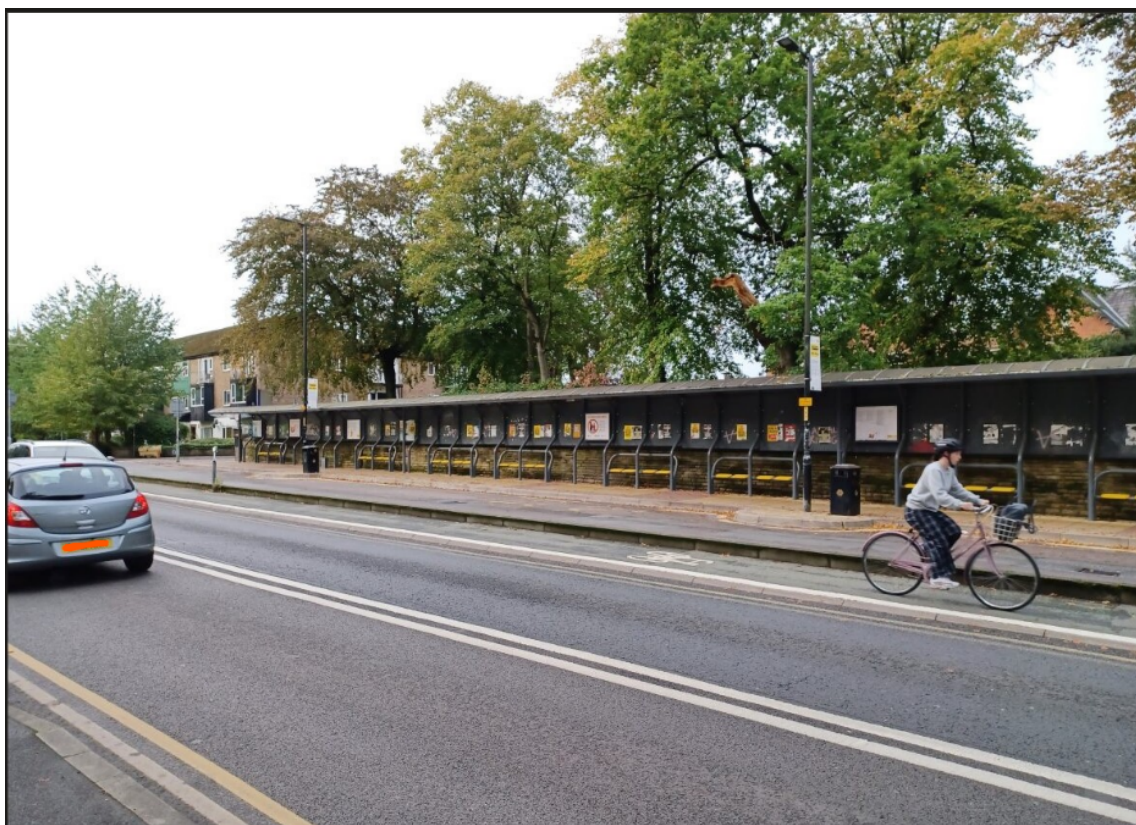
Existing northbound bus stop on Wilmslow Road opposite main entrance into the Campus
