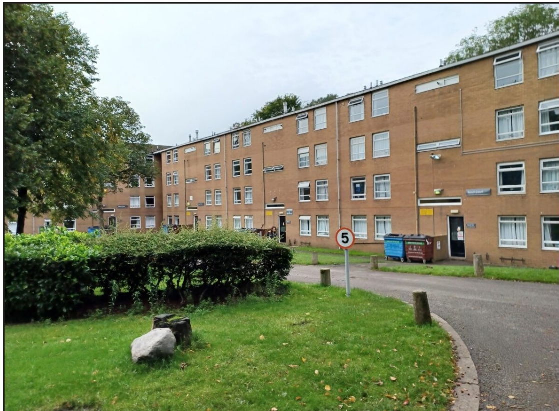
Existing Campus Building (Beech Court)
